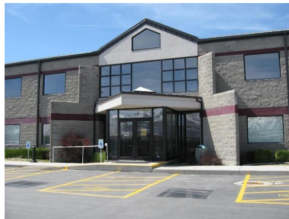
Figure 7: The front entrance to the UTA Paratransit Evaluation Center
